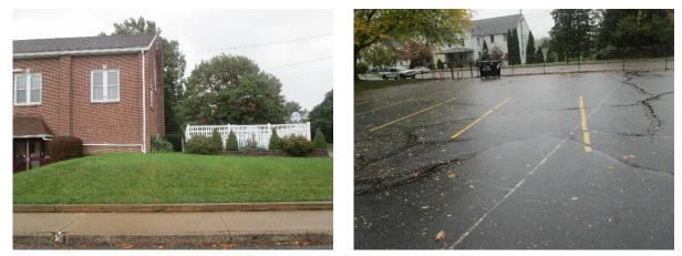
Parking spots to the south of the building can be replaced with porous asphalt to capture and infiltrate stormwater. Installing a rain garden adjacent to the building can capture, treat, and infiltrate roof runoff. A preliminary soil assessment suggests that the soils have suitable drainage characteristics for green infrastructure.
