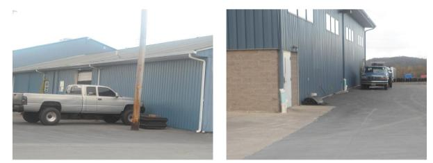
Parking spots can be replaced with porous asphalt to capture and infiltrate stormwater. Installing a cistern will capture roof runoff and provide water for washing vehicles or other non-potable uses. A preliminary soil assessment suggests that the soils have suitable drainage characteristics for green infrastructure.
