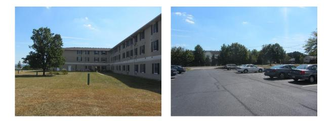
Parking spots to the west of the building can be replaced with porous asphalt to capture and infiltrate stormwater. Rain gardens adjacent to the building can capture, treat, and infiltrate roof runoff. A preliminary soil assessment suggests that the soils have suitable drainage characteristics for green infrastructure.
